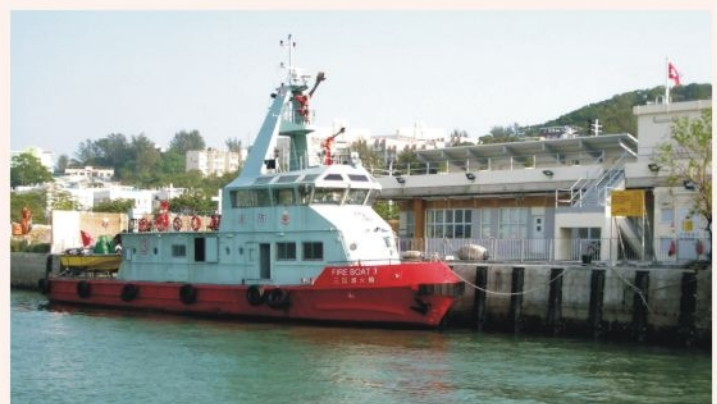
● 長洲滅火輪消防局投入服務 The newly commissioned Cheung Chau Fireboat Station
